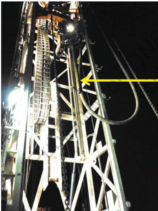
Joint remaining in elevators
