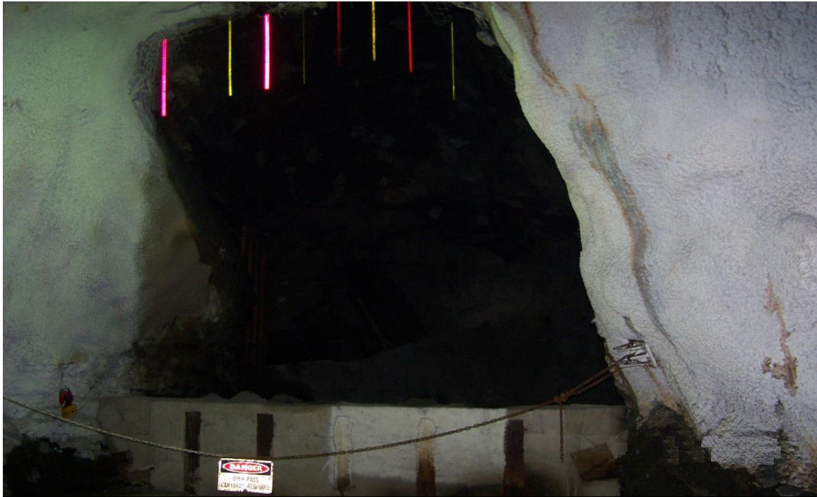
Figure 1: Example of a permanent stop log
