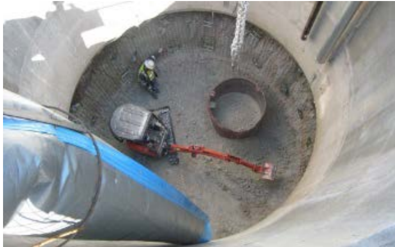
Example of an excavator in use during a shaft sink
